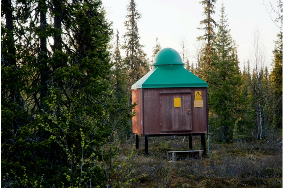
Figure 37, The ALIS station in Tjautjas. The glass dome in the ceiling, holding a camera, is dismantled during summer season as there is too much light for the Aurora Borealis.
