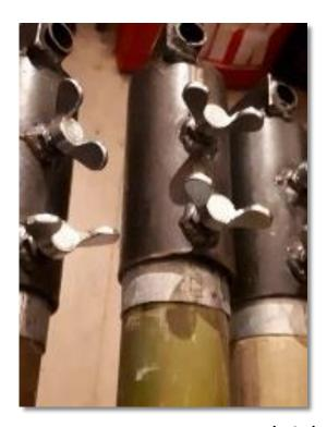
New way to connect and tighten the connection with the bamboo so it cannot move anymore
