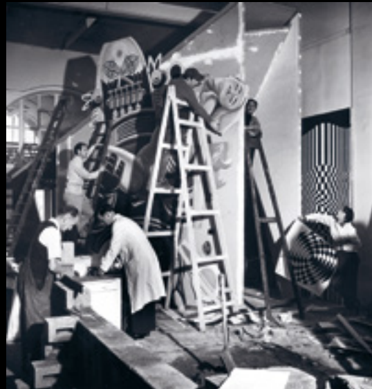
37 The Group 2 show, created by Richard Hamilton, John McHale and John Voelcker, is installed at the exhibition This is Tomorrow at the Whitechapel Art Gallery, London, 1956.
