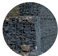
6. Rubble gabion line foundation
