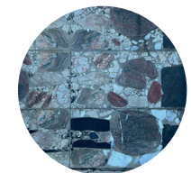
10. Large rubble concrete walls (load bearing)
