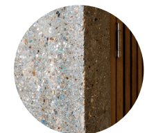
7. Rubble aggregate foundation
