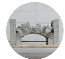
15.1 Parallel flat sided rubble vaulted roof
