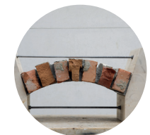
15.3 Reclaimed brick vaulted slab
