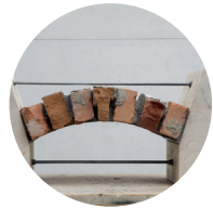
15.3 Reclaimed brick vaulted slab
