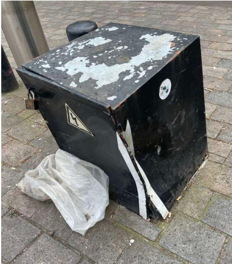
Electrical box (Crushed), Den Haag, 2024
